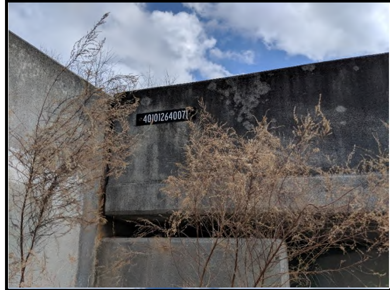
2 The bridge is identified as structure # 401012640071.
